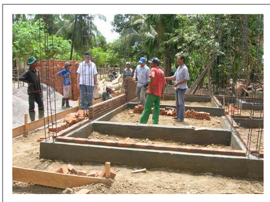
Photo: An UMCOR house under construction in Bireuen, Indonesia. Credit: UMCOR
